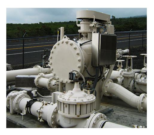
**Electricity from water treatment:** This 45-kilowatt turbine, installed in a water treatment plant in Hawaii, pulls double duty: It generates electricity while also reducing water pressure in pipes leading from higher elevations to a storage tank.
